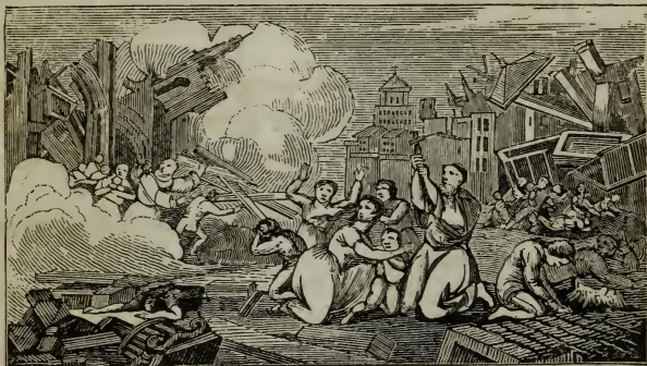
Earthquake at Lisbon.
